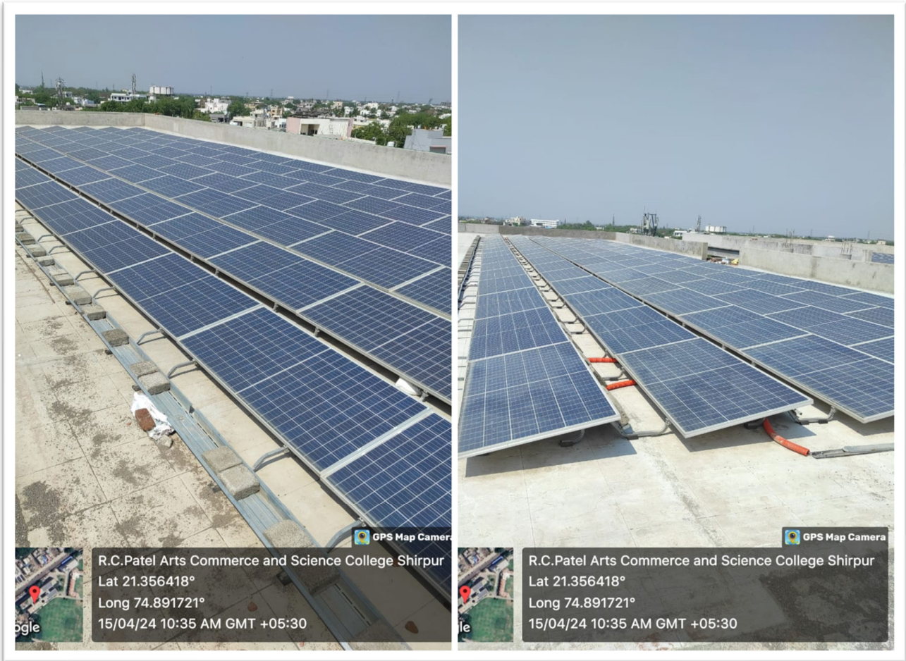
Solar Panels Unit 1 – On Grid – Output 32kw
