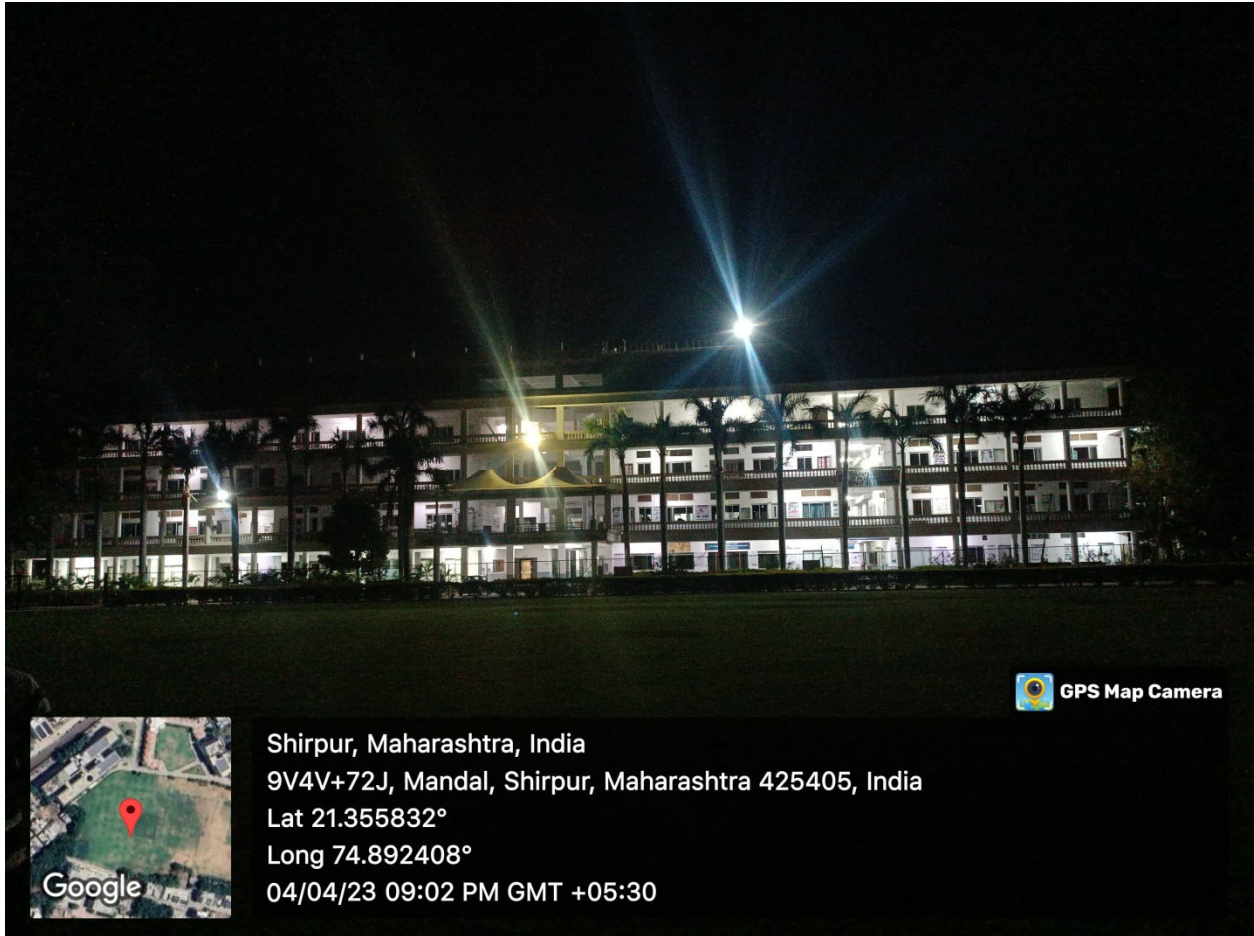
Figure 4 Use of LED Bulbs 01
