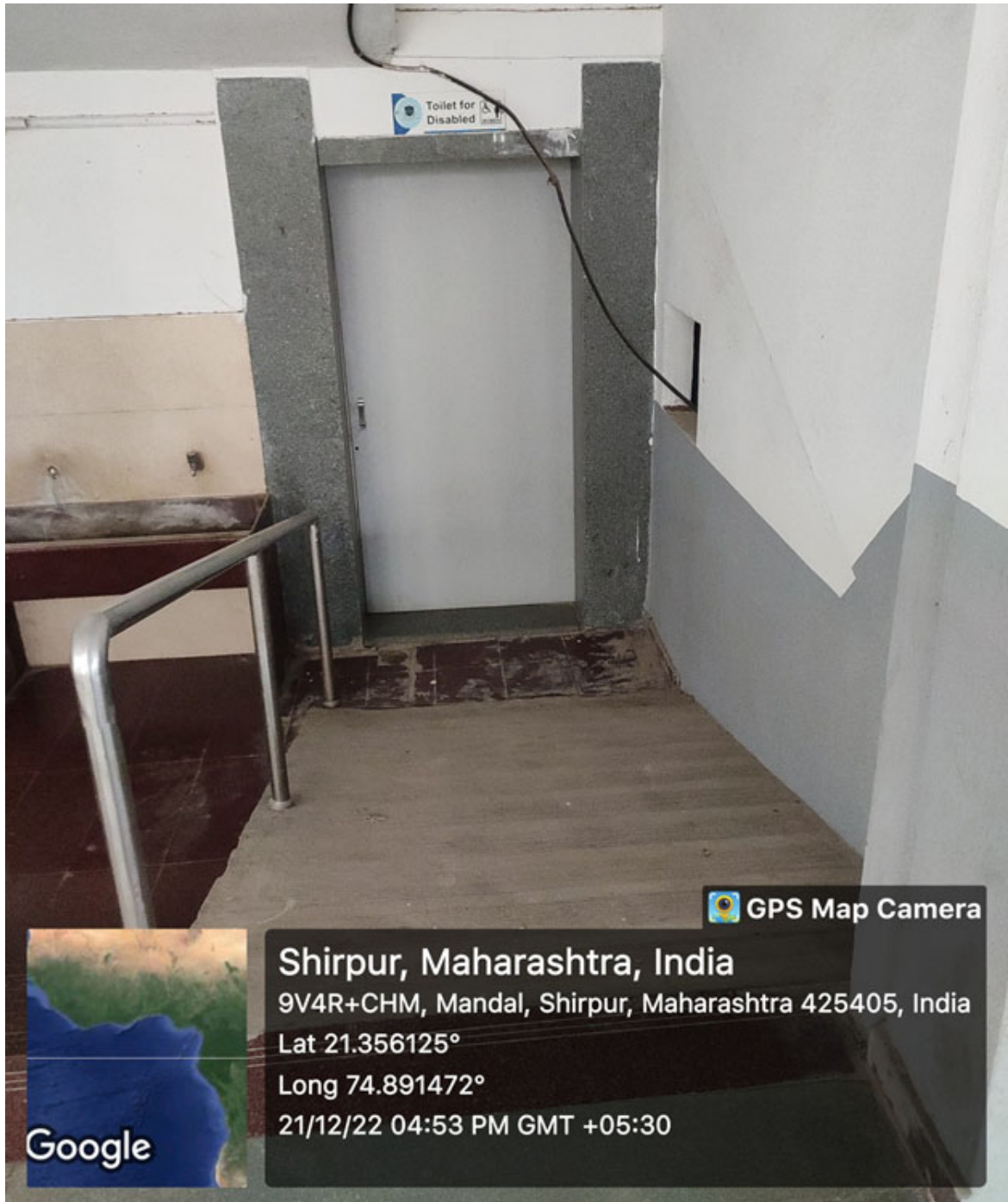
Figure 38 Disabled Friendly Washroom
